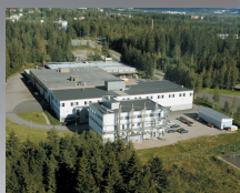
奥林芬兰总部拉赫蒂工厂 Oilon Headquarters in Lahti, Finland
